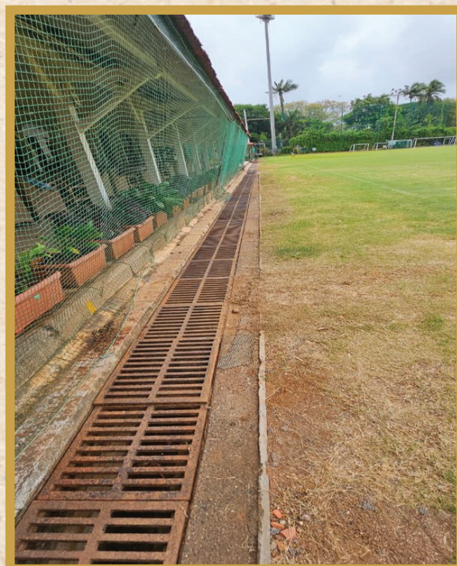
❖ Resolved water stagnation issue by providing a proper drainage slope .
